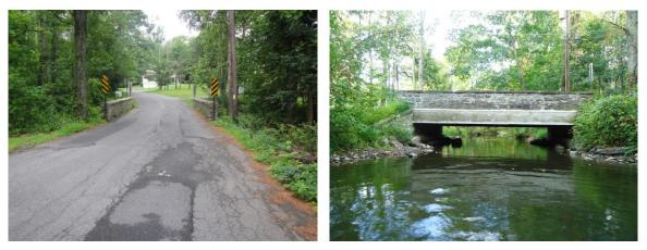
Figure 1. Photographs of the downstream Aspinwall Road Bridge. The relatively narrow bridge opening and limited vertical clearance constrict streamflow during high flow conditions.
