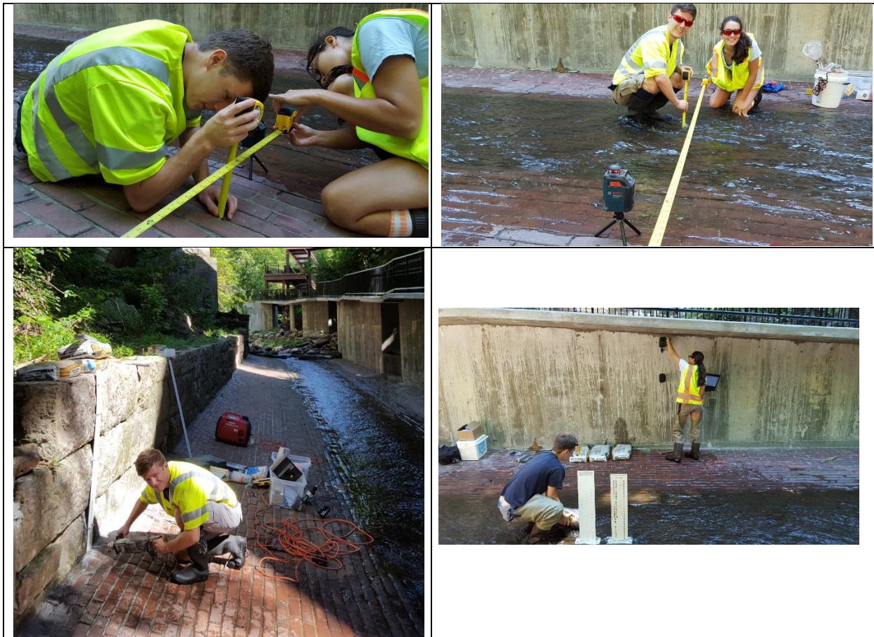
Figure 3: Building and calibrating the stream gauge. a) Measuring the geometry of the race in depth vs linear distance from the stone wall and separately, the depth vs. the brick row locations. b) A laser level was used to determine depth c) a third depth gauge sign was mounted on the north stone wall. d) Cameras are mounted on south side concrete wall pointing toward two depth measurement signs.
