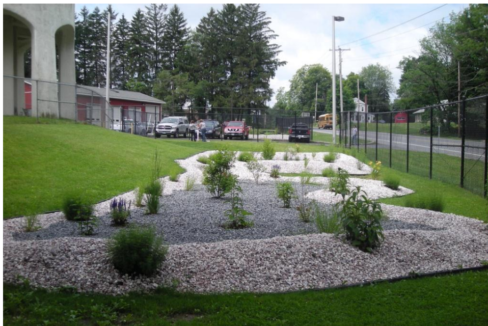
Figure 11. Rain gardens at the City of Newburgh Water Treatment Plant (Photo courtesy K. Sumner, 2009).
