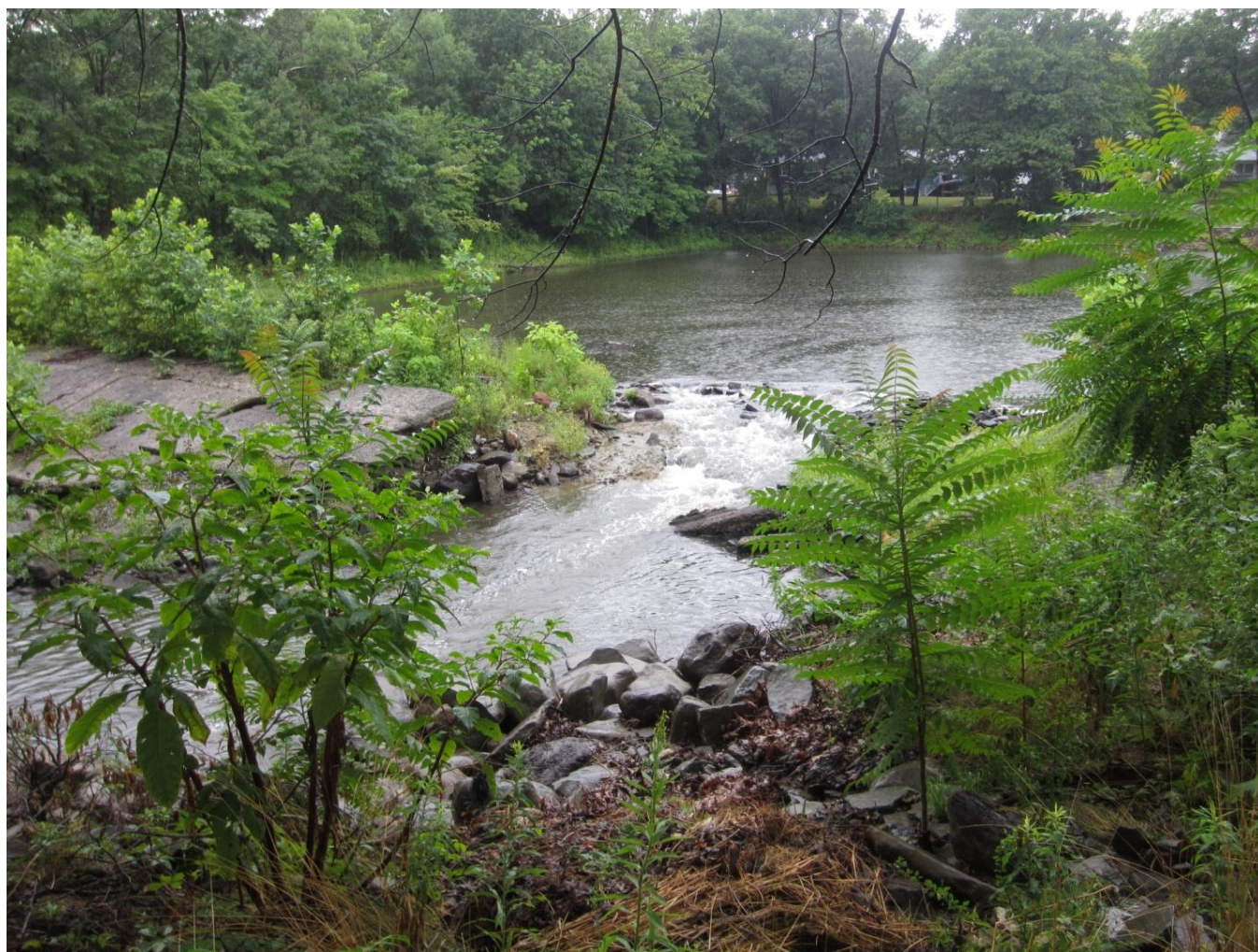
Figure 6. Winona Lake Dam breach, July 2012.
