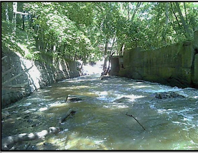
Figure 25. Looking downstream from Holden Dam at confined stream channel of Lower Quassaick Creek.
