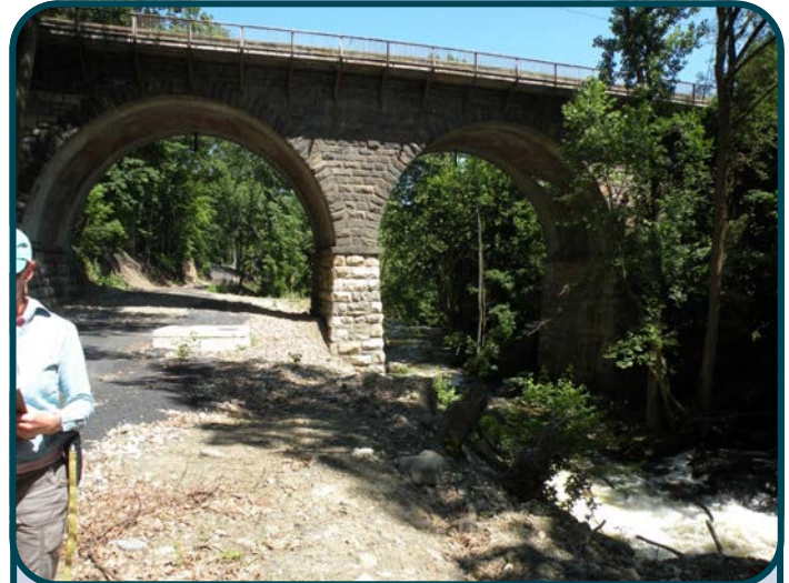
Photo 1: Shown is the Mill Street Bridge with Quassaick Creek flowing on the right and construction road, which could potentially serve as a public trail, on the left.
