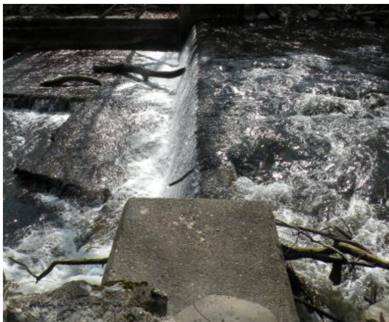
Figure 10. Low-head impoundment at the American Felt and Filter Site on the Quassaick Creek. Photo courtesy P. Smith, 2012.
