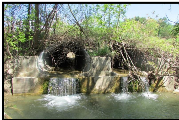
Culverts such as this one constrict the natural flow of the stream, have a perched outlet that only strong swimmers can jump and contain no natural streambed. Many culverts and dams fragment stream habitats.
