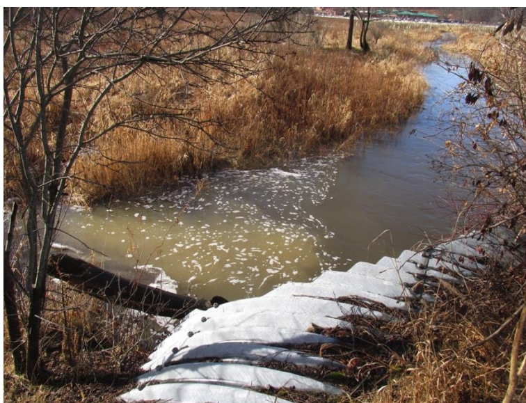
Figure 17. A nearby construction site causes a silt plume in a tributary of the Monhagen Brook in 2018. The site had erosion and sediment control measures in place, but they were not installed properly.
