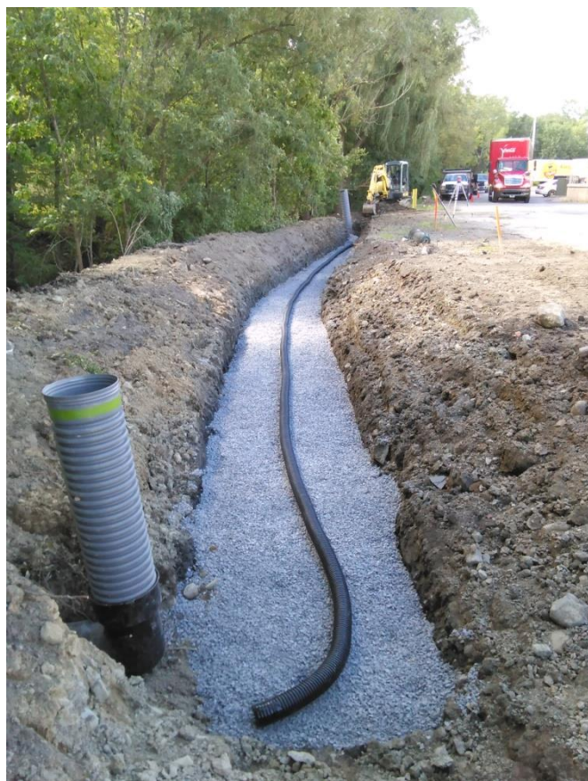
Figure 28. Construction of the Campbell Plaza Bioretention Basin
