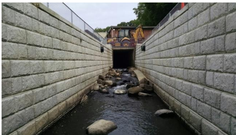
Figure 19. This section of the Brook east of Monhagen Avenue in Middletown “daylights” for a short run before returning underground. The pre-cast concrete block walls typify the extension of grey infrastructure techniques beyond the streets, catch basins, and collection systems to the stream itself.
