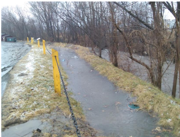
Figure 20. Parking lot runoff is collected and treated by this Bioretention Basin retrofit in the City of Middletown. Before the retrofit, the runoff drained directly into the Monhagen Brook, seen in the right of the photo. Measures such as this can be expected to remove about 40% of the phosphorus from the runoff stream. Similar removal rates can be expected for other dissolved pollutants.
