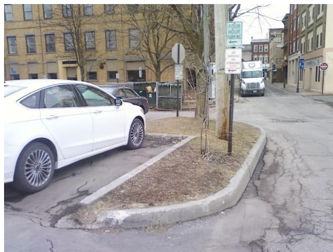
Figure 27. Parking lot islands, like this one in the James Street parking lot, will be depressed below rather than elevated above the adjacent pavement when the lot is retrofitted. Runoff from the pavement will then flow into the island and be cleansed and filtered by soil and vegetation. The dumpsters in the background have already been relocated from the parking lot.
