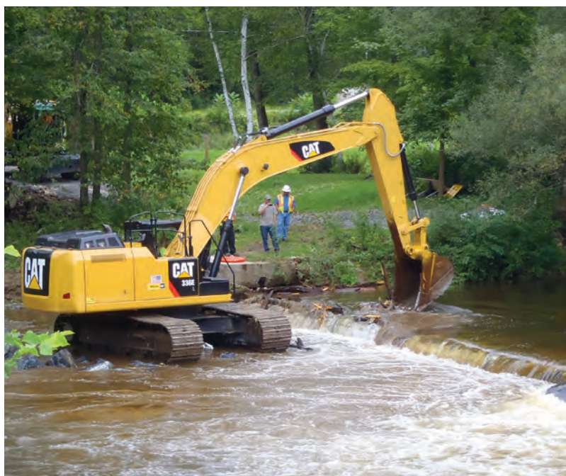
Henry Bridge Dam removal, North Pownal, Vermont
