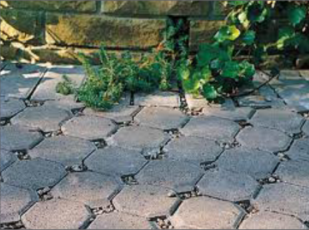
Permeable interlocking concrete pavers
