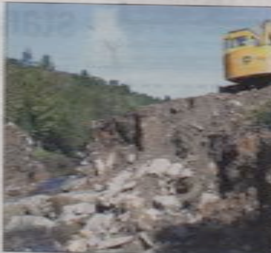
Water from the 11-acre lake at Mountaindale Park in Fallsburg drains through a gaping hole in the 38-year-old dam.
