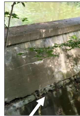
Spalling and Cracking
