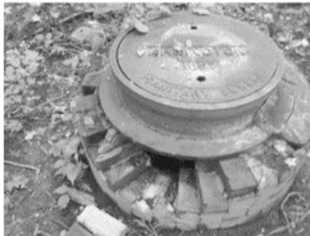
Fig. 23: Decaying sewage infrastructure is a source of fecal contamination to the stream. This vault on the Vassar College campus was replaced in spring 2008.
