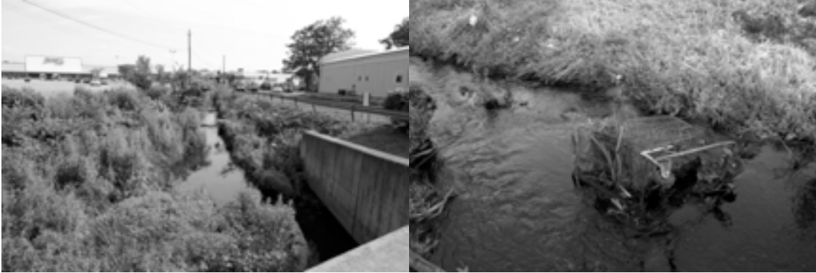
Fig. 7: Photos of the Casperkill channel in the Dutchess and 44 Plaza area. The stream has been artificially straightened and deepened and lined with rock cobble rip-rap. Trash, including shopping carts, plastic bags, fast-food wrappers, and soda bottles, litters the site.
