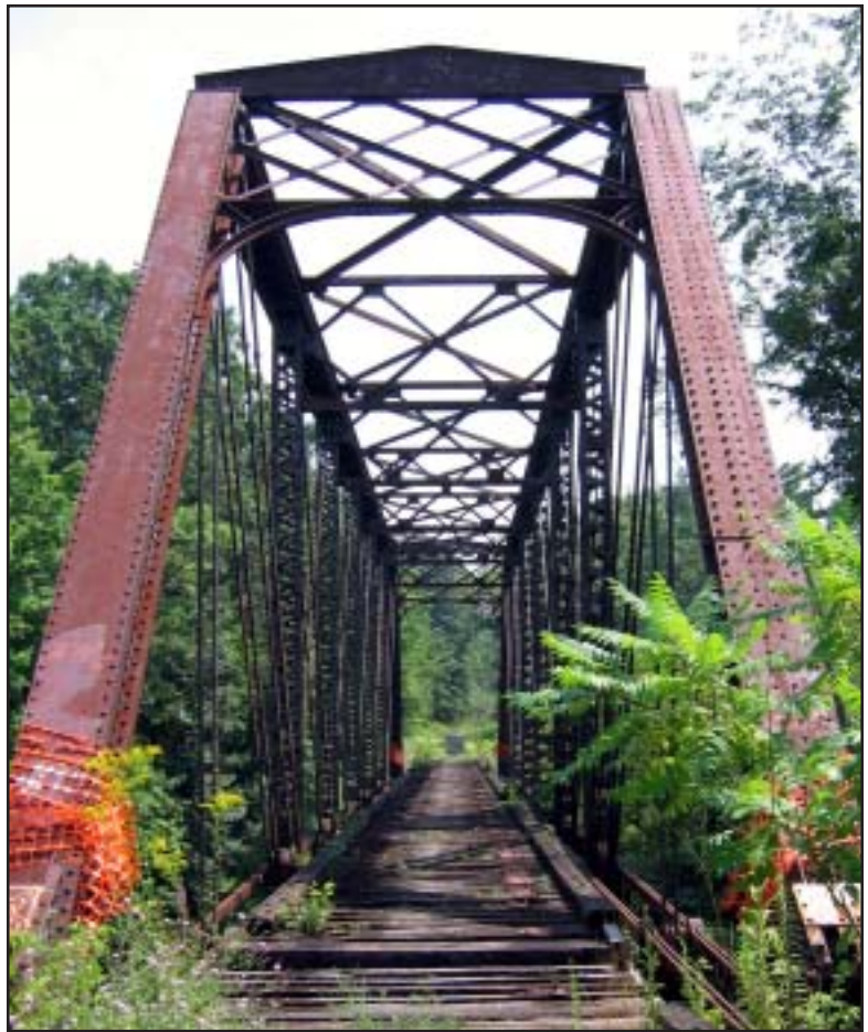
Iron and steel truss railroad bridge over the Normans Kill
