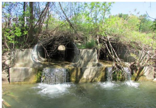
Figure 1: Culverts such as this one constrict the natural flow of the stream and contain no natural streambed substrate. Perched culverts such as this one fragment stream habitats.
